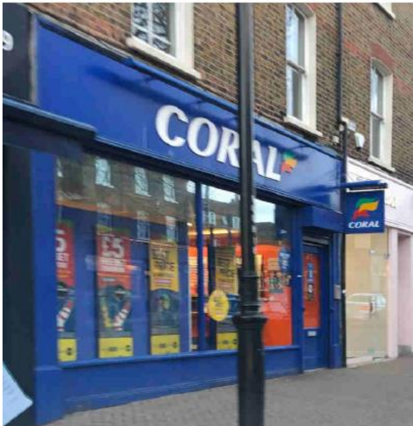
Figure 2: Pre-Existing Shop Front
